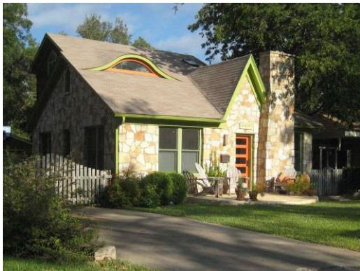
The roof has been raised slightly and a dormer window added to accommodate the addition, while maintaining the original roof form and scale of the building.
