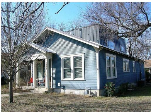
The addition is set forward flush with the front façade of the original building. The flat roof is not compatible with the character of the original building. Modern or Contemporary design may be appropriate for an addition, provided that it is not visible from the right-of-way.
