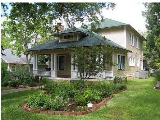
The addition is set back from the front façade and mirrors the roof form of the original building.
